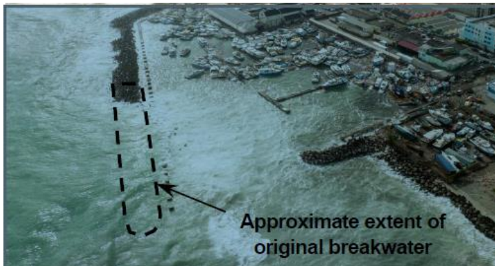
Figure 3: Breakwater Post Hurricane Beryl
