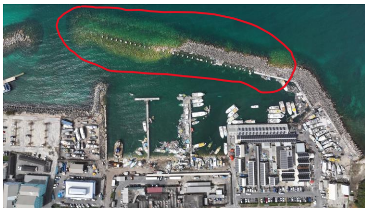
Figure 1: Marina and Breakwater damaged during Hurricane Beryl
